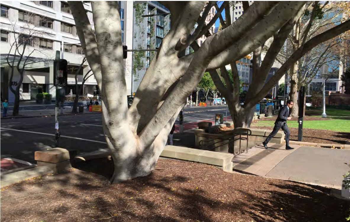
The widened access to the Park off the Liverpool Street entry will require the removal of the two Fig Trees either side of the existing steps. The sandstone walls and copes will also need to be dismantled.
